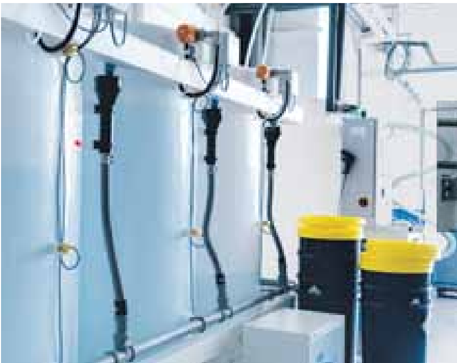
▲ Granumixplus machine to produce dialysis concentrate in the clinic: The prepared concentrate is transferred directly to the dedicated tank for storage. Thanks to this closed system, the concentrate stays clean and dust-free without spilling.
